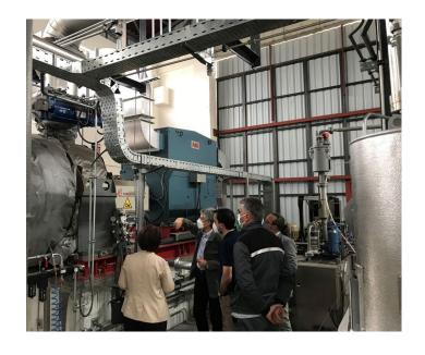
heat sources. Hot water is generated, and in typical processes this is then cooled down. But UNIDO has supported BGB to utilize this hot water to produce more thermal energy. The plant has installed an economizer and heat transfer network that moves this thermal energy back to the pellet production system to power the drying process and to broiler farms for heating.
