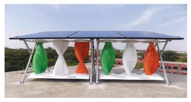
Figure 47: Solar wind hybrid system
