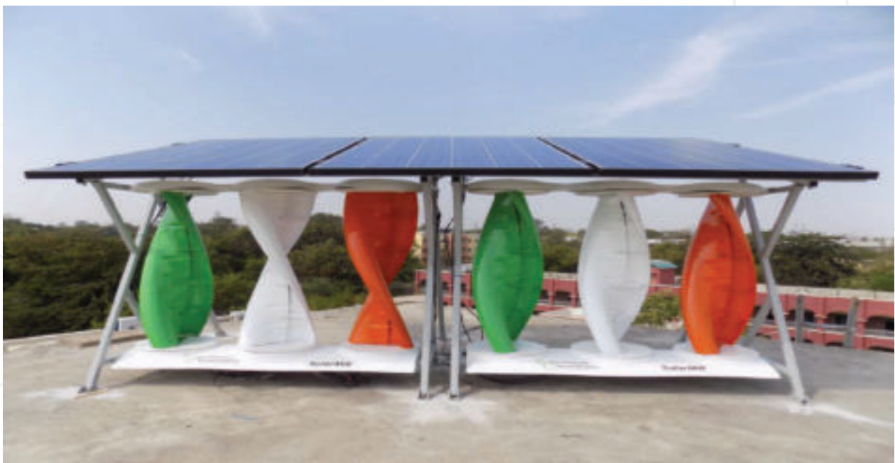
Figure 32: Solar wind hybrid system
