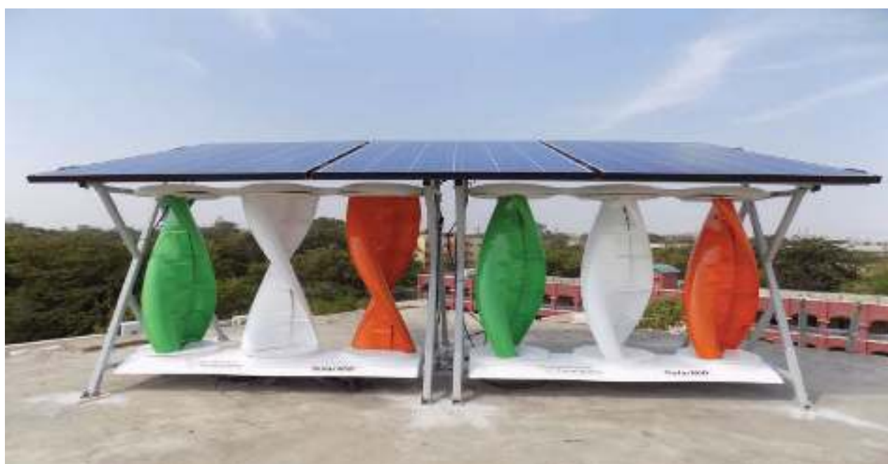
Figure 51: Solar wind hybrid system
