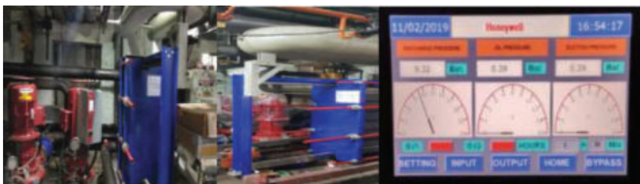
Figure 25: Post Implementation – Direct Cooling Method
