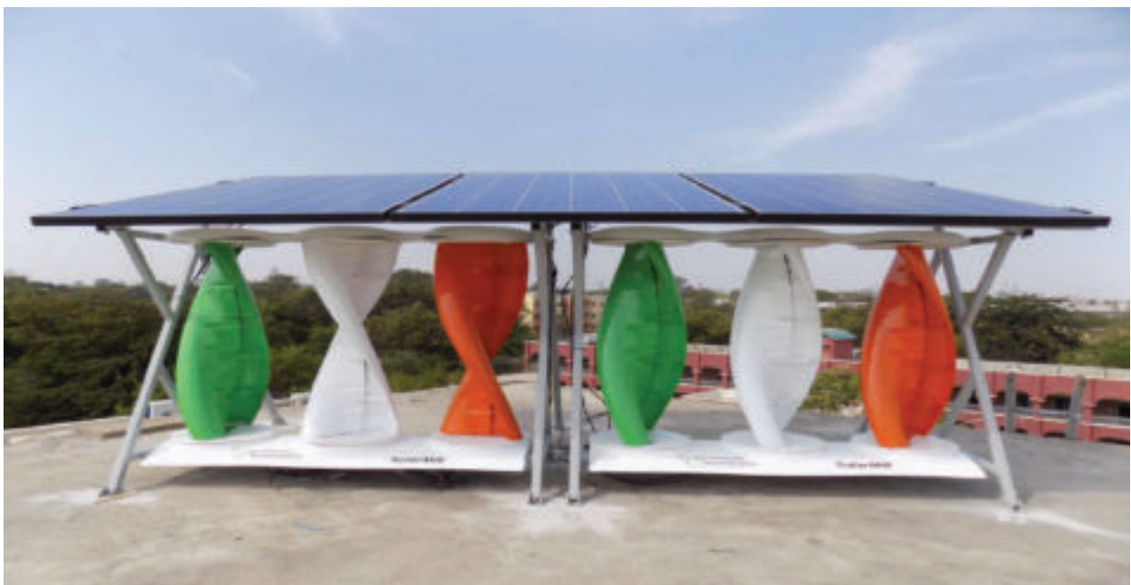
Figure 50: Solar wind hybrid system
