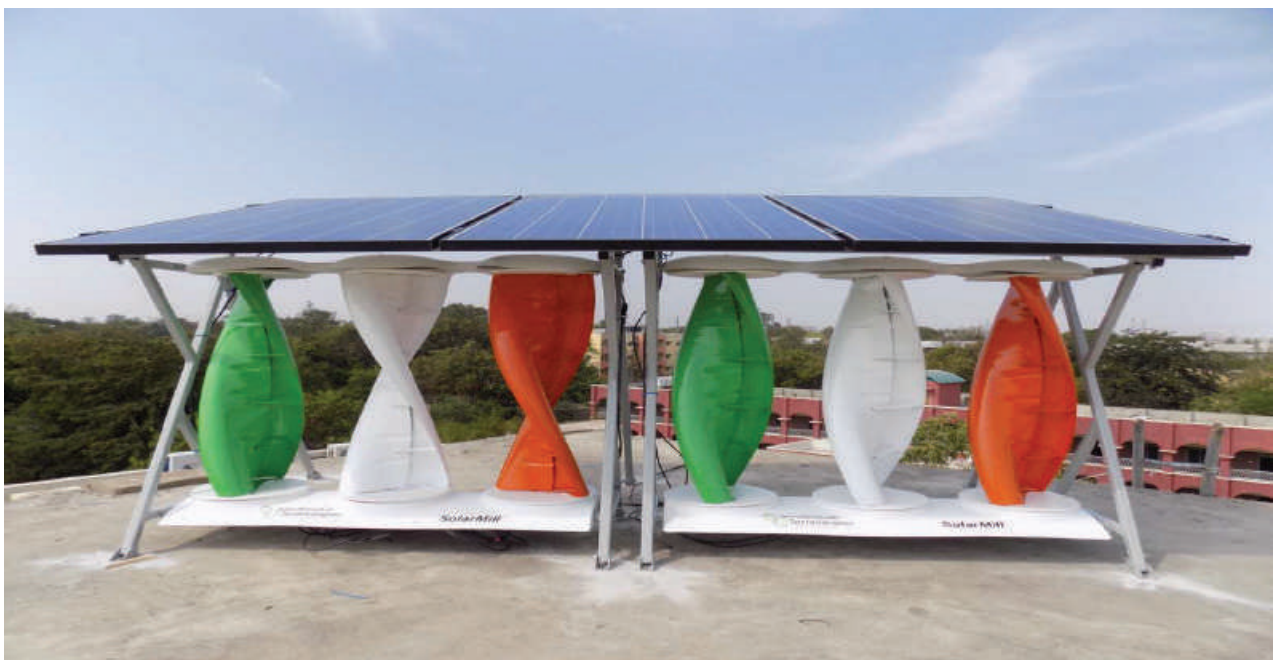
Figure 51: Solar Wind Hybrid System
