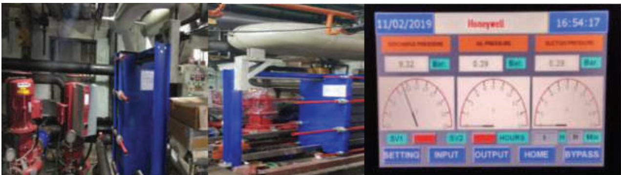
Figure 26: Post Implementation – Direct Cooling Method
