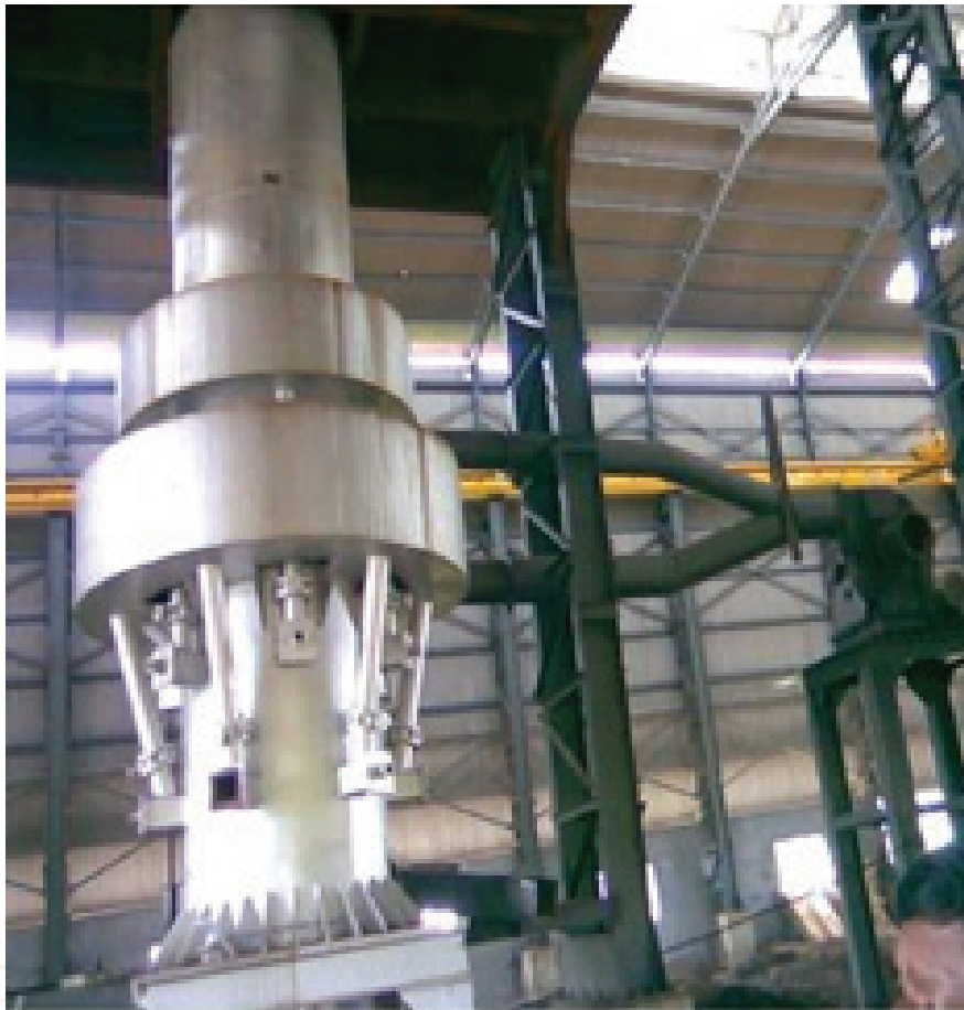
Figure 11: Divided Blast Cupola
