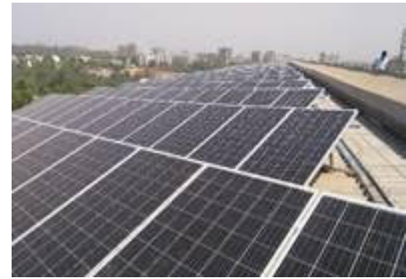
Figure 20: Solar PV Installation
