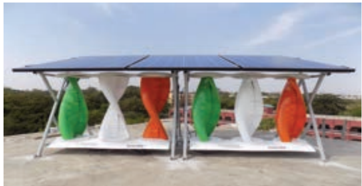
Figure 22: Solar Wind Hybrid System
