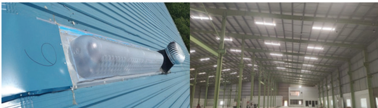
Figure 30: Light Pipe Installation
