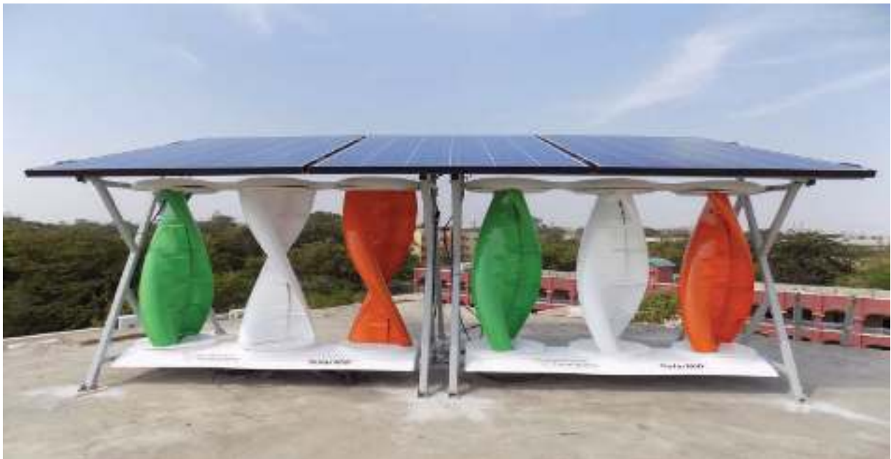
Figure 50: Solar wind hybrid system
