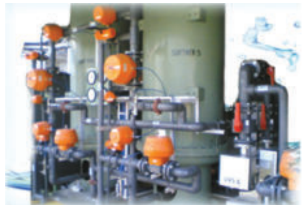
Figure 51: Water softener unit
