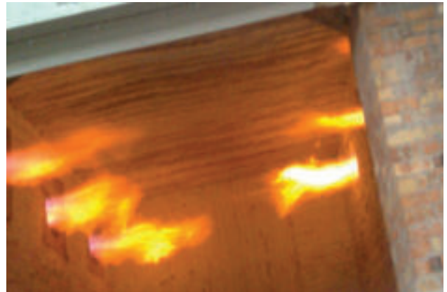
Figure 50: Improper air to fuel ratio
