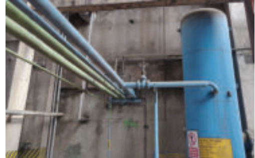
Figure 31: Existing compressed air piping
