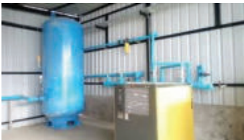
Figure 32: HDPE Aluminium Pipe line
