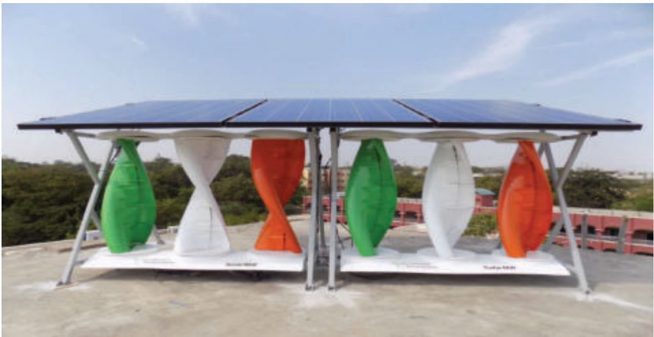
Figure 43: Solar wind hybrid system
