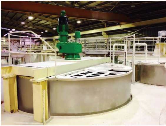
Figure 6: Slurry agitation and storage
