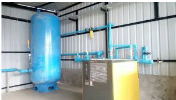
Figure 47: HDPE Aluminium Pipe-line
