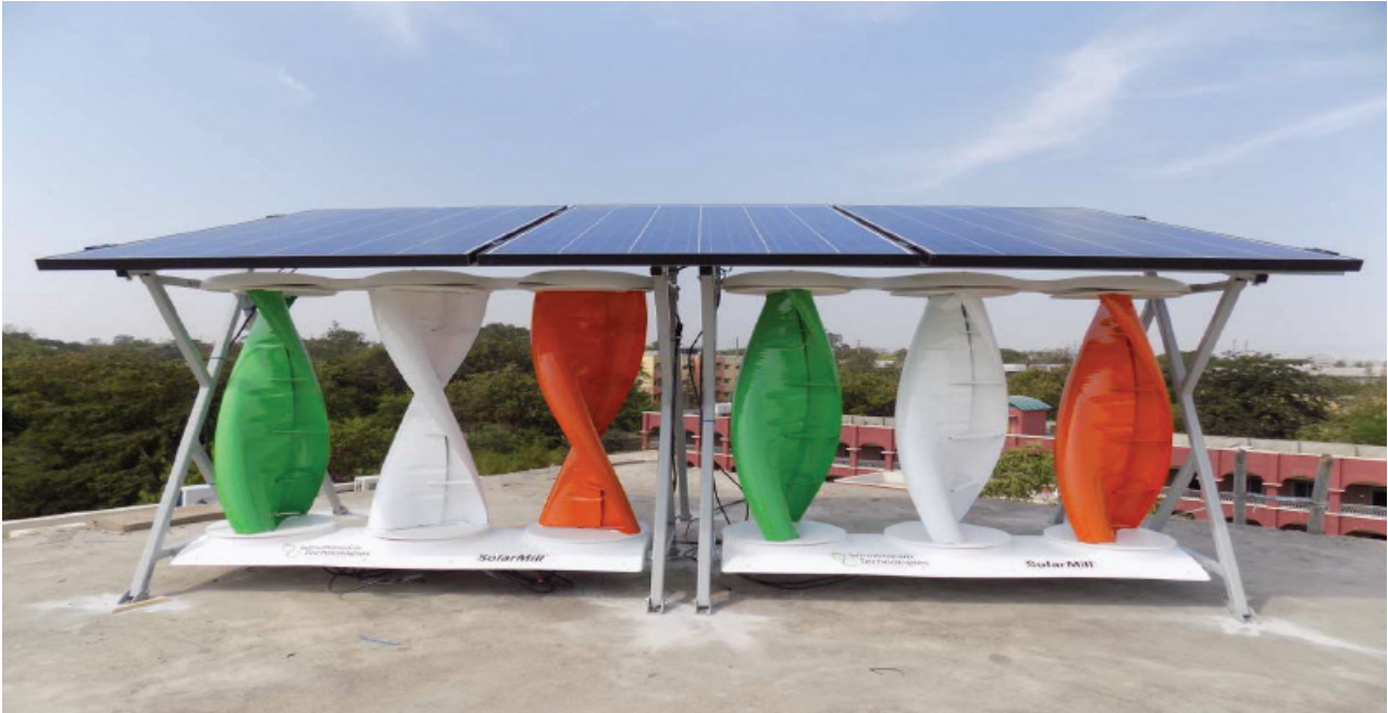
Figure 58: Solar wind hybrid system
