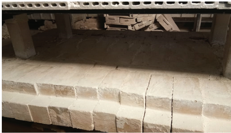
Figure 33: Existing high thermal mass refractory in kiln car
