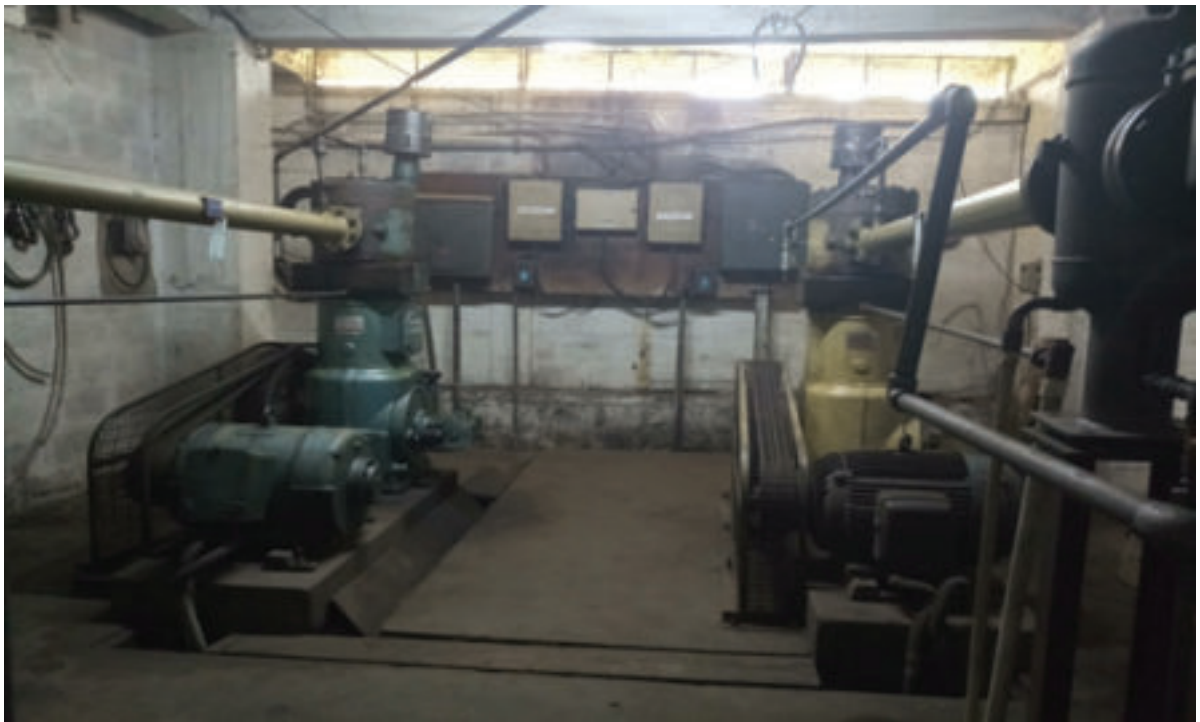
Figure 27: Old reciprocating compressor
