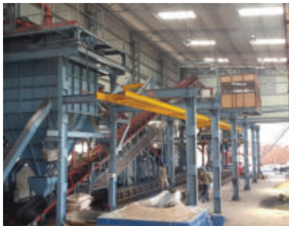
Figure 39: Energy efficient sand plant
