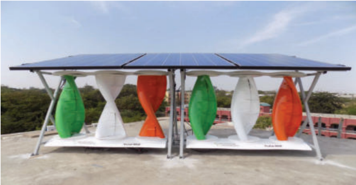
Figure 52: Solar-wind hybrid system
