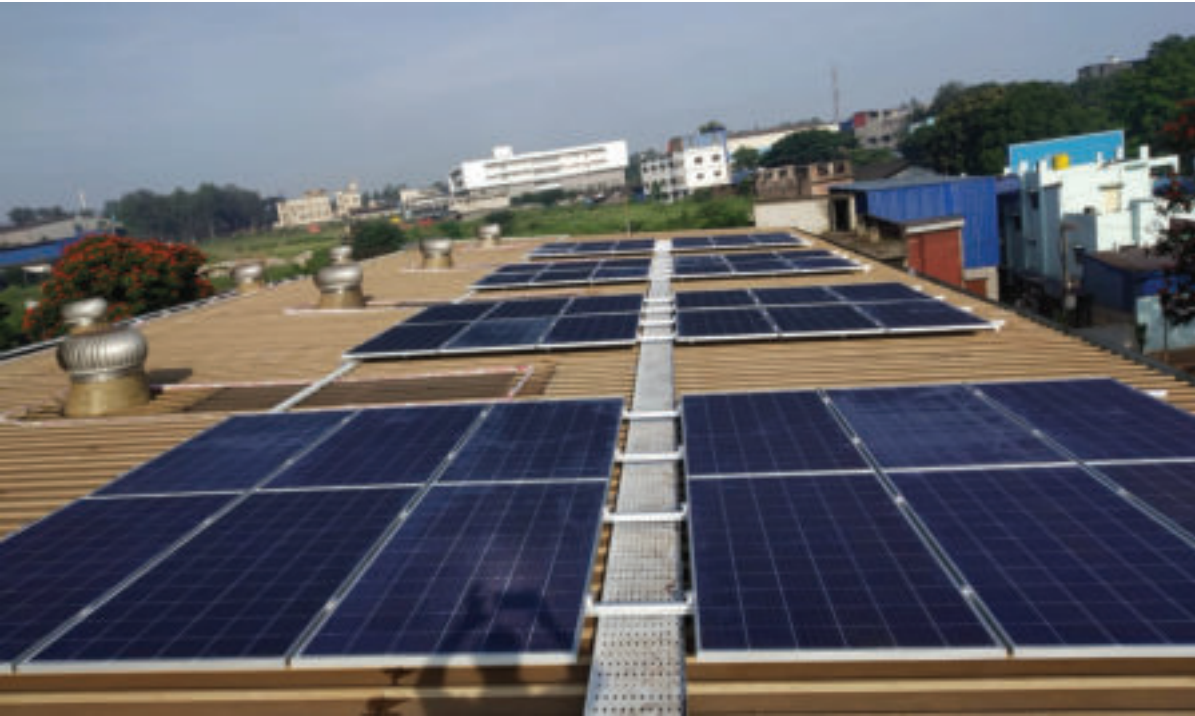
Figure 48: Rooftop solar PV system
