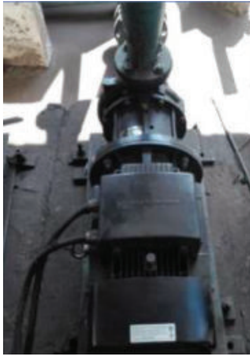
Figure 25: New pump photo and specifications
