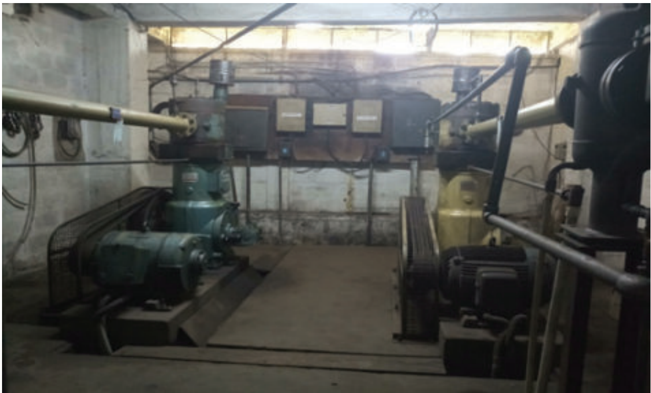
Figure 27: Old reciprocating compressor
