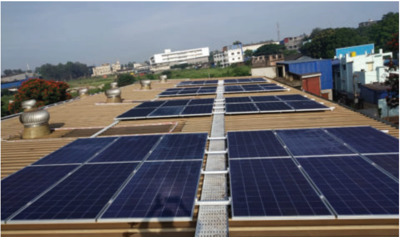
Figure 51: Rooftop solar PV system
