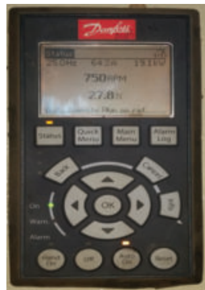
Figure 32: VFD panel of compressor
