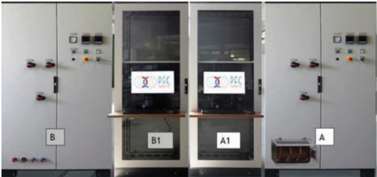
Figure 35: Reactive current injection system installed in main panel
