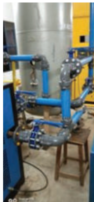
Figure 48: Aluminium pipeline for compressed air
