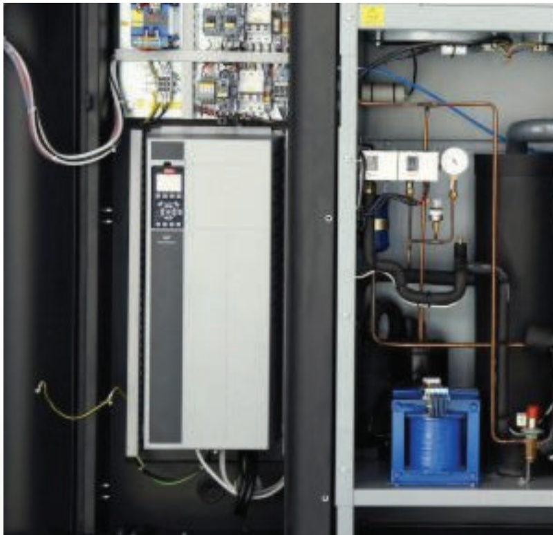
Figure 39: VFD installed in the panel of a compressor
