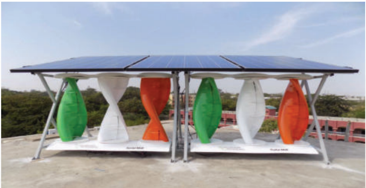
Figure 53: Solar-wind hybrid system
