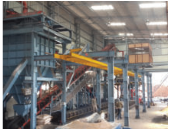
Figure 43: Energy efficient sand plant
