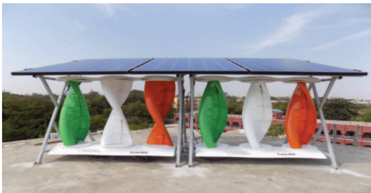
Figure 52: Solar wind hybrid system
