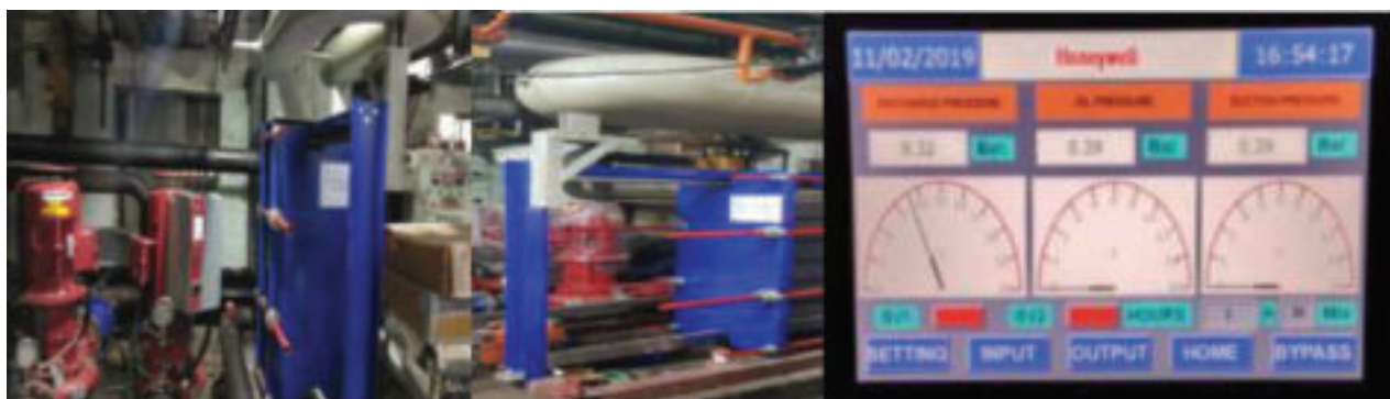
Figure 27: Post Implementation – Direct Cooling Method
