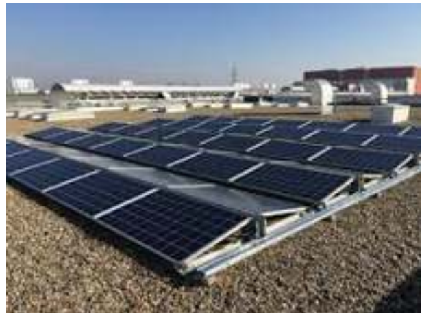
Figure 21 : Solar PV installation
