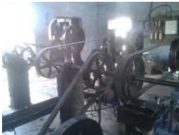
Figure 24: Inefficient belt and pulley drives
