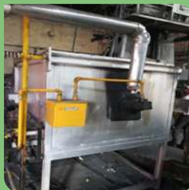
Energy Efficient LPG Fired Forging Furnace in Victor Forging
