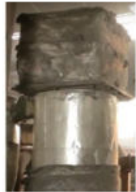
Figure 13: Radiative cum convective recuperator
