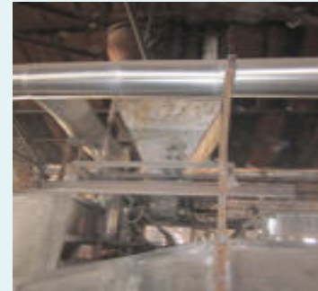
Modified pulverized coal feeding system at TK Steel
