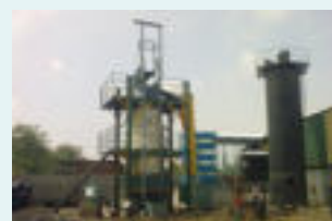
Biomass based producer gas plant
