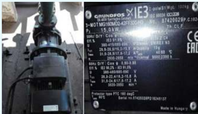
New EE Pump at Integra Automation
