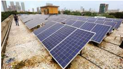
Figure 15: Roof Top Solar PV Installation
