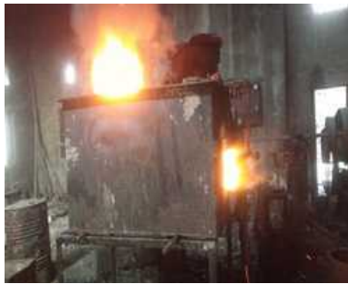
Figure 4: Typical FO fired forging furnace
