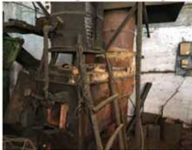
Figure 7: An oil fired forging furnace
