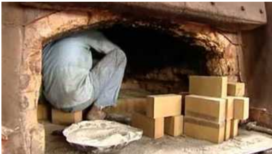
Figure 21: Heat treatment furnace veneering process
