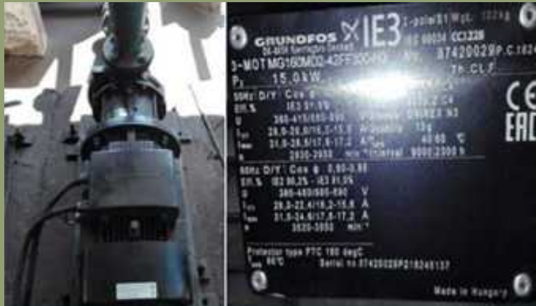
New EE Pump at Integra Automation
