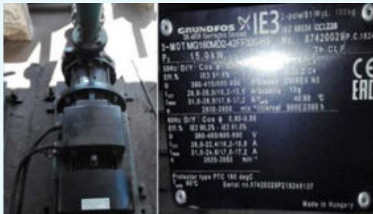
New EE Pump at Integra Automation
