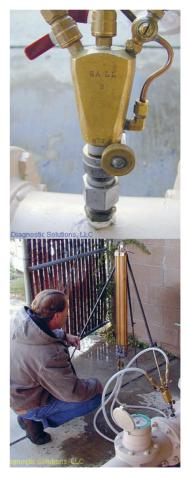
Fig. 12.21. Flow Reading with a Multi-port Pitot Tube
