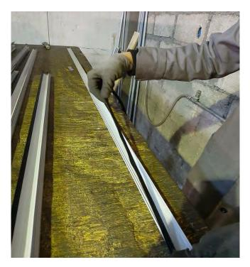
Figure 113 Rubber sealing fixation [3]
