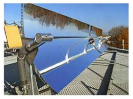
Figure 15 Parabolic trough collector, NEP
